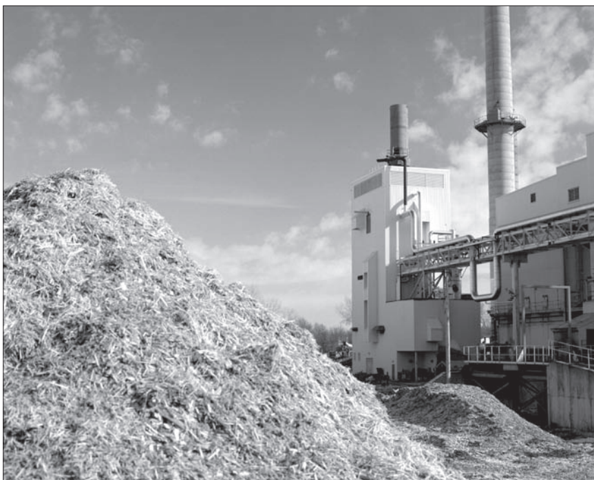
LANDFILL GAS INTO ELECTRICITY This small power plant located at a landfill produces low cost, reliable electricity.
